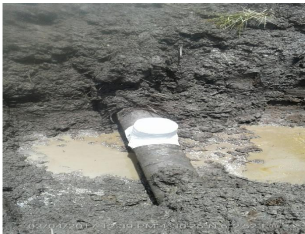
FIGURE: 3 REPAIR WORK
